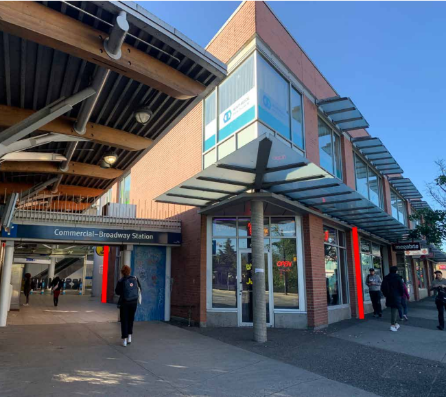
Commercial Drive Storefront #2
